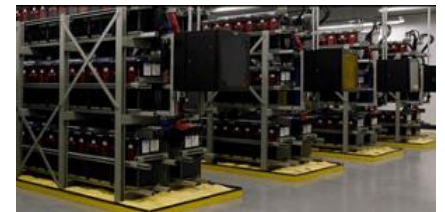
Figure 4.13 Battery Bank
