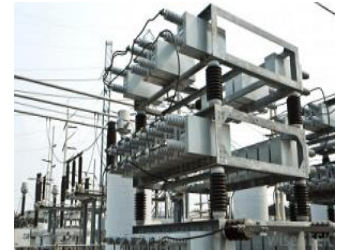
Figure 4.12 Capacitor Bank
