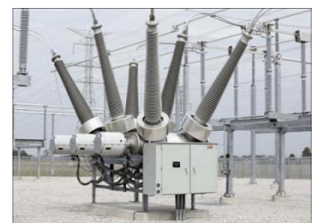
Figure 4.10 Circuit Breaker
