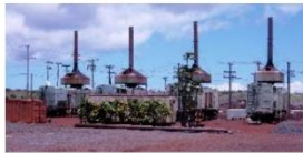
(6) 1.0 MW EMD Diesel Generators (2) 2.2 MW Caterpillar Diesel
